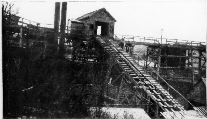
Incline from Quarry to Trestle Passing Over the Tops of the Kilns
